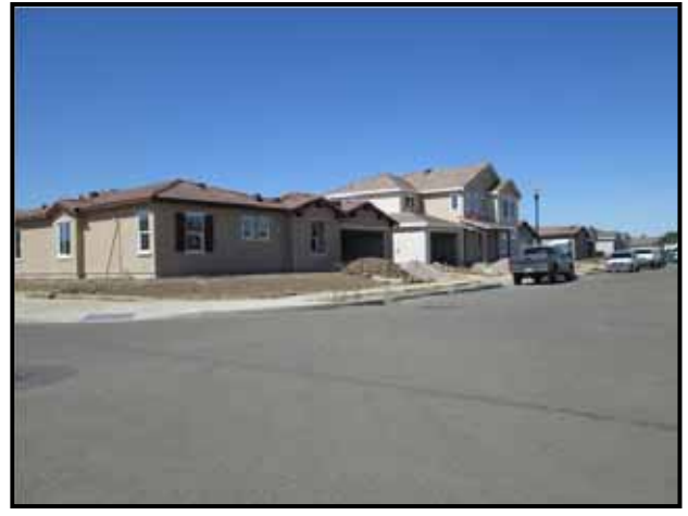
Southwesterly view from Stratford Way Lots under construction
