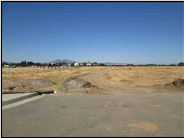
Westerly view from Grain Parkway Partially finished lots
