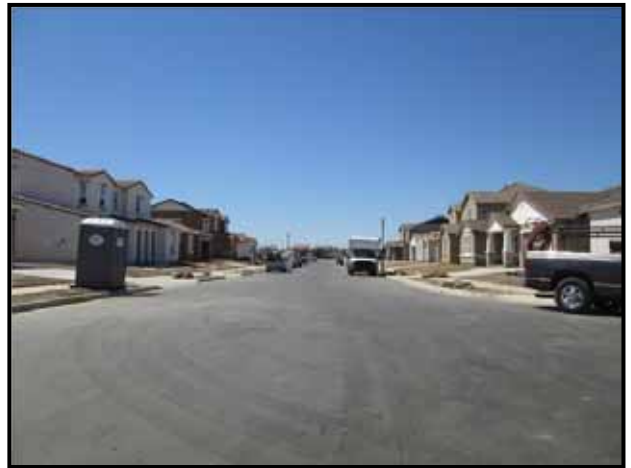
Southerly view from Bellerose Court Lots under construction
