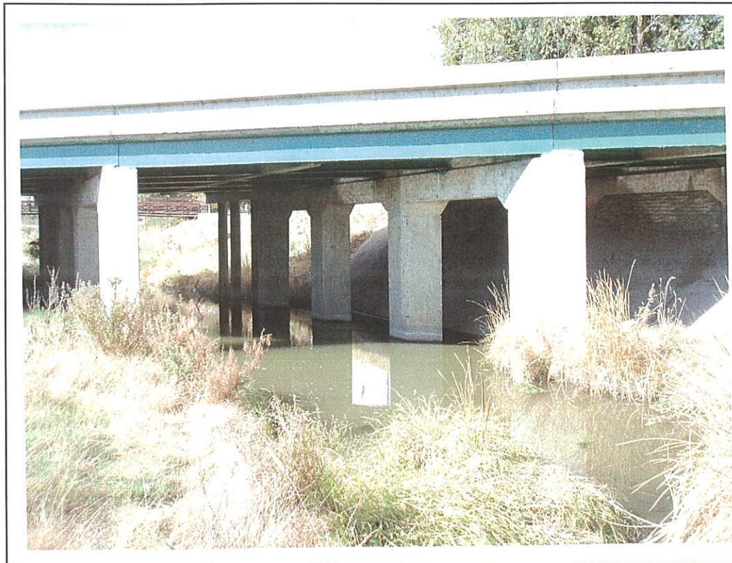
Brentwood Boulevard bridge at Marsh Creek, looking northeast (downstream); 10/9/07.
