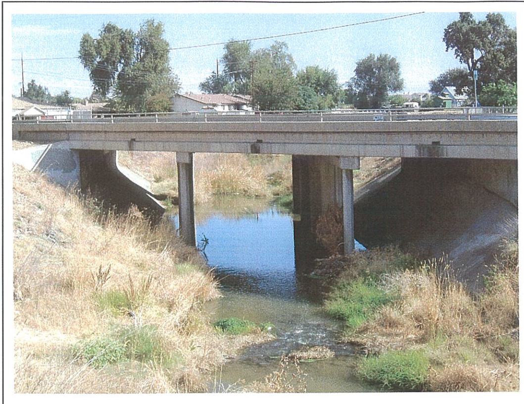
Brentwood Boulevard bridge at Marsh Creek, looking southwest (upstream); 10/9/07.
