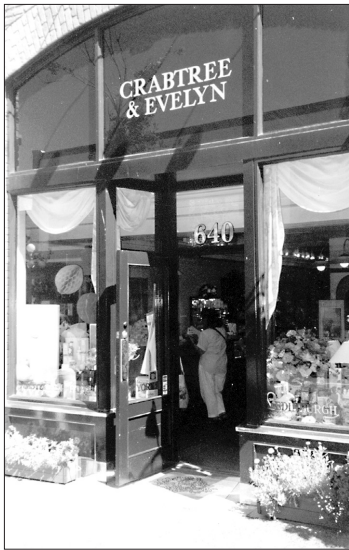
Bulkhead with moulding and planters
