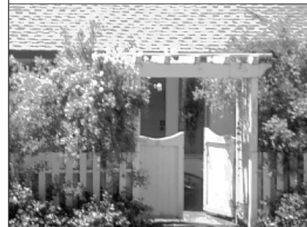
Picket fencing and front entry gate/trellis with flowering plants maintain a residential style and character
