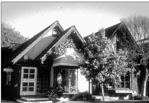
Example of contemporary building with residential scale and character
