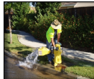
Hydrant Flushing
