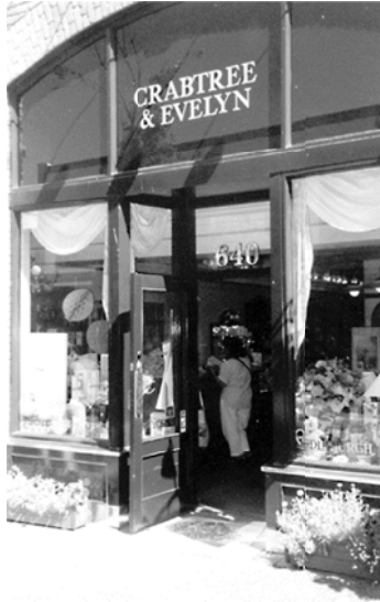
Bulkhead with moulding and planters
