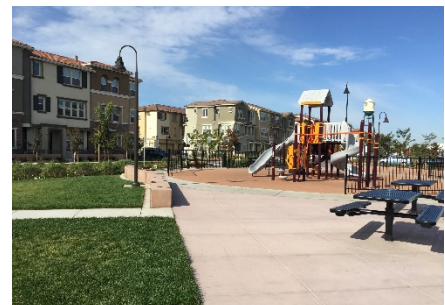
In multi-family residential developments, dwelling units or amenity areas should be sited adjacent to the common open space areas that incorporate playgrounds and parkland.
