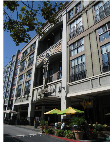
Designs should utilize architectural elements to enhance building facades. These include cornices, lintels, sills, and balconies.
