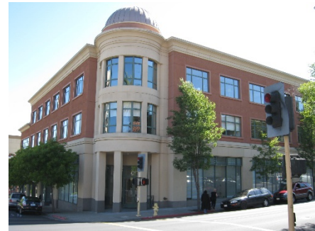
Buildings, incorporating special architectural and building design features, shall be placed on street corners to acknowledge the prominence of the corner.
