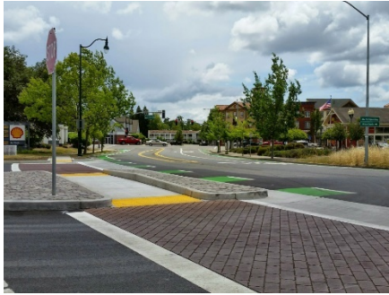
Intersection with pedestrian refuge, enhanced crosswalk markings, and green bike lanes
