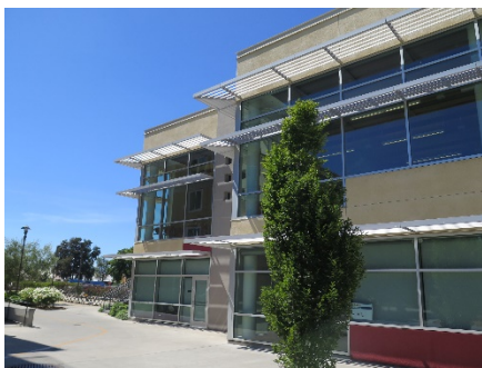
To maximize natural lighting on south-facing facades, light shelves should be provided on windows.
