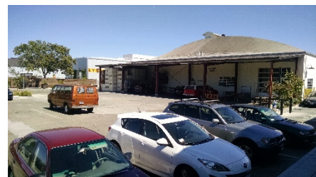
Loading docks and service areas, and parking, wherever possible, shall be located behind buildings.
