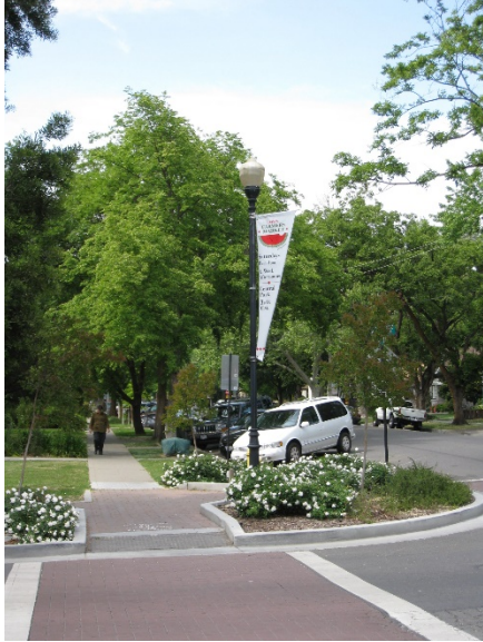
To make pedestrian crossings as safe as possible, construct bulbouts and distinguish the crossing area with differentiated pavement.
