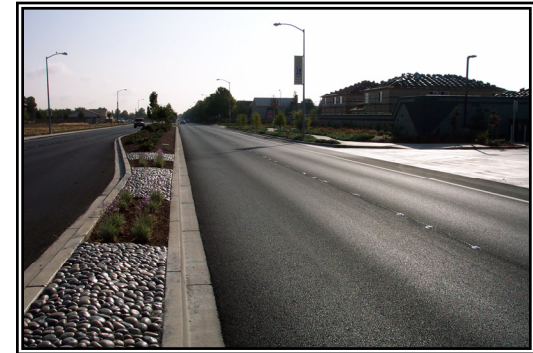
Balfour Road Overlay Project
