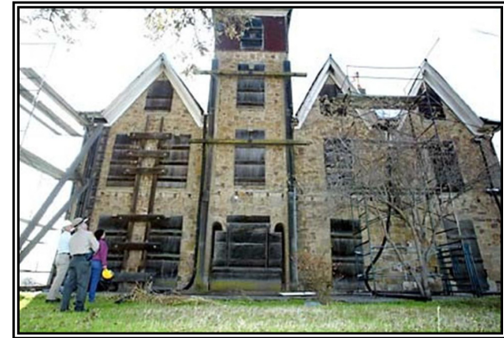
John Marsh House Restoration
