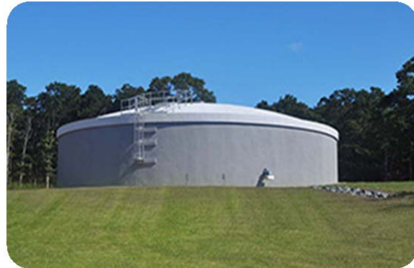
Non-Potable Storage Facility
