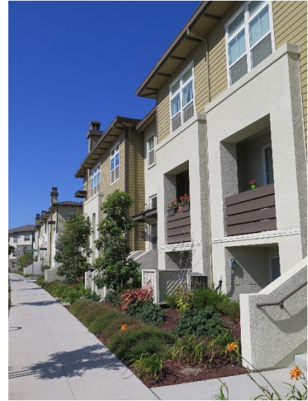
For multi-family residential development, setback areas shall be landscaped to establish transition zones between the sidewalk and street-level residential units and entries.
