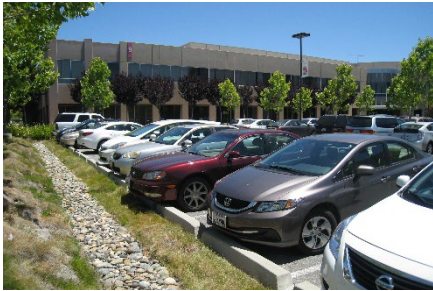
Reduce stormwater runoff by implementing features that promote groundwater infiltration, such as bioswales.
