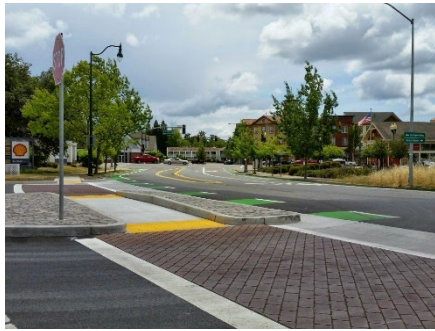
Intersection with pedestrian refuge, enhanced crosswalk markings, and green bike lanes
