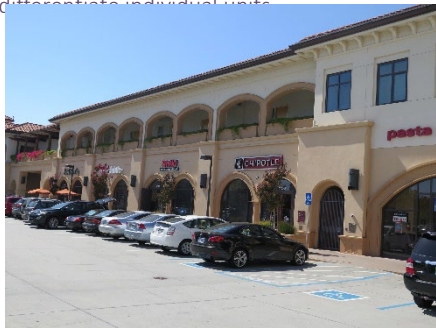
Commercial developments should incorporate animating features, such as arcades, display windows, and entry areas, along front facades and side facades that face a public right-of-way.
