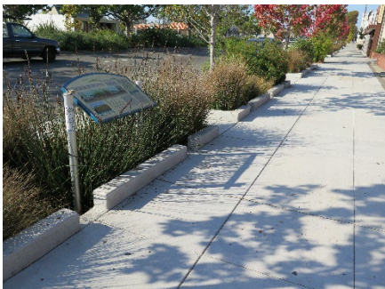
Install naturally drained, landscaped stormwater planters including along sidewalks. Install educational and interpretive signage along the planters.
