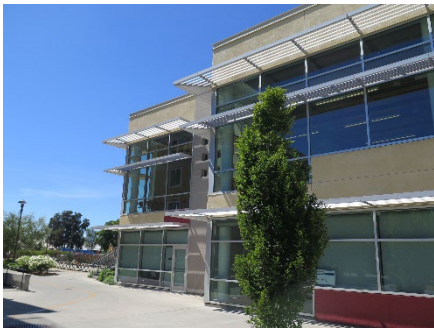
To maximize natural lighting on south-facing facades, light shelves should be provided on windows.
