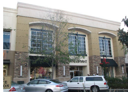
Transparent windows, storefronts, show windows, building entries, dwelling entries, and other active uses shall be placed along street and public open space frontages. Designs should differentiate between the amount of the façade reserved for fenestration for the street-level and upper stories.
