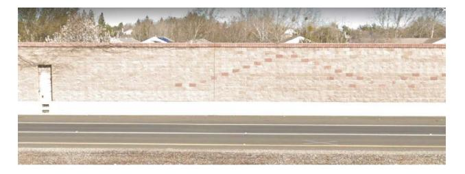
At the time of the Route 4 Bypass construction, it should have been apparent that the raised elevation of Route 4 (i.e., future development) was incompatible with the existing soundwall height of the Siena community (i.e., existing development).
